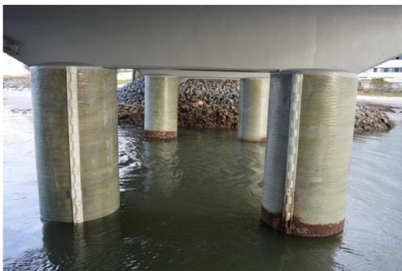
A three-year collaborative development project between Joinlox and USQ resulted in the development and commercialisation of a new type of composite pile repair system made of a prefabricated fibre-reinforced polymer (FRP) jacket with an innovative joining system for infrastructure rehabilitation.
